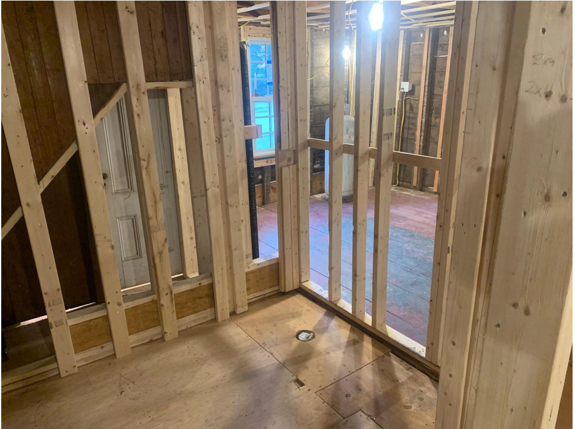
Inside – Level 2 – First Floor – ADA Compliant Restroom 2
