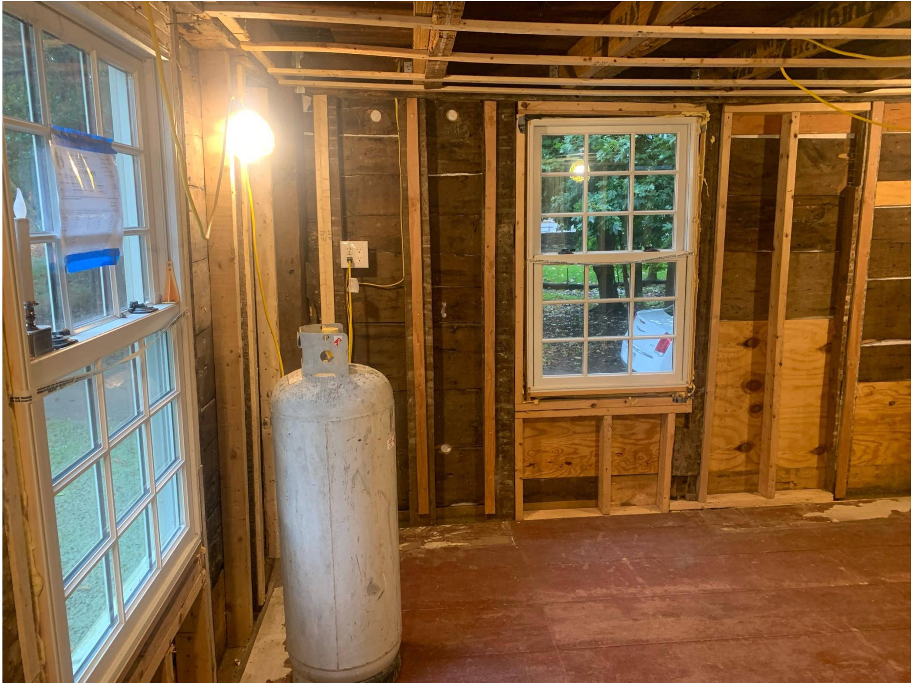
Inside – Level 2 – First Floor CollecUons Room
