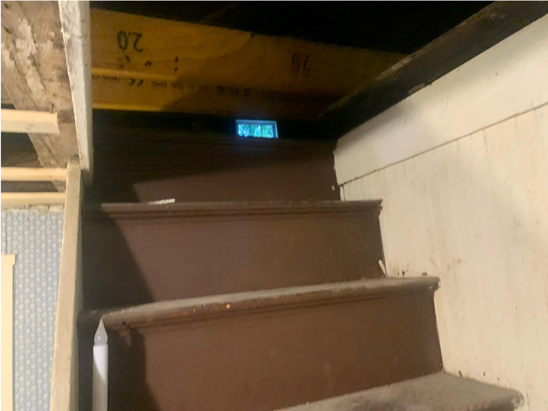
Inside – Level 4 – AZc Floor Stairs
