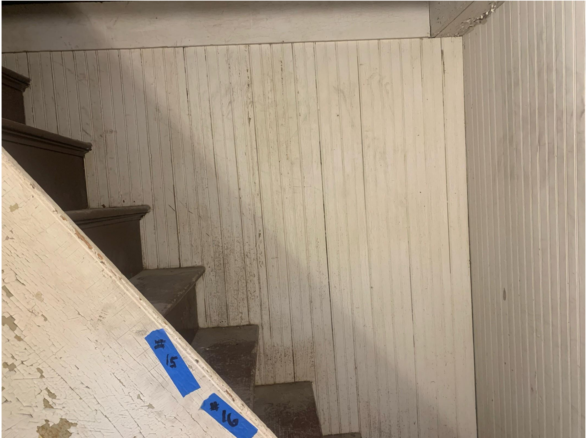
Inside – Level 4 – AZc Floor Stairs
