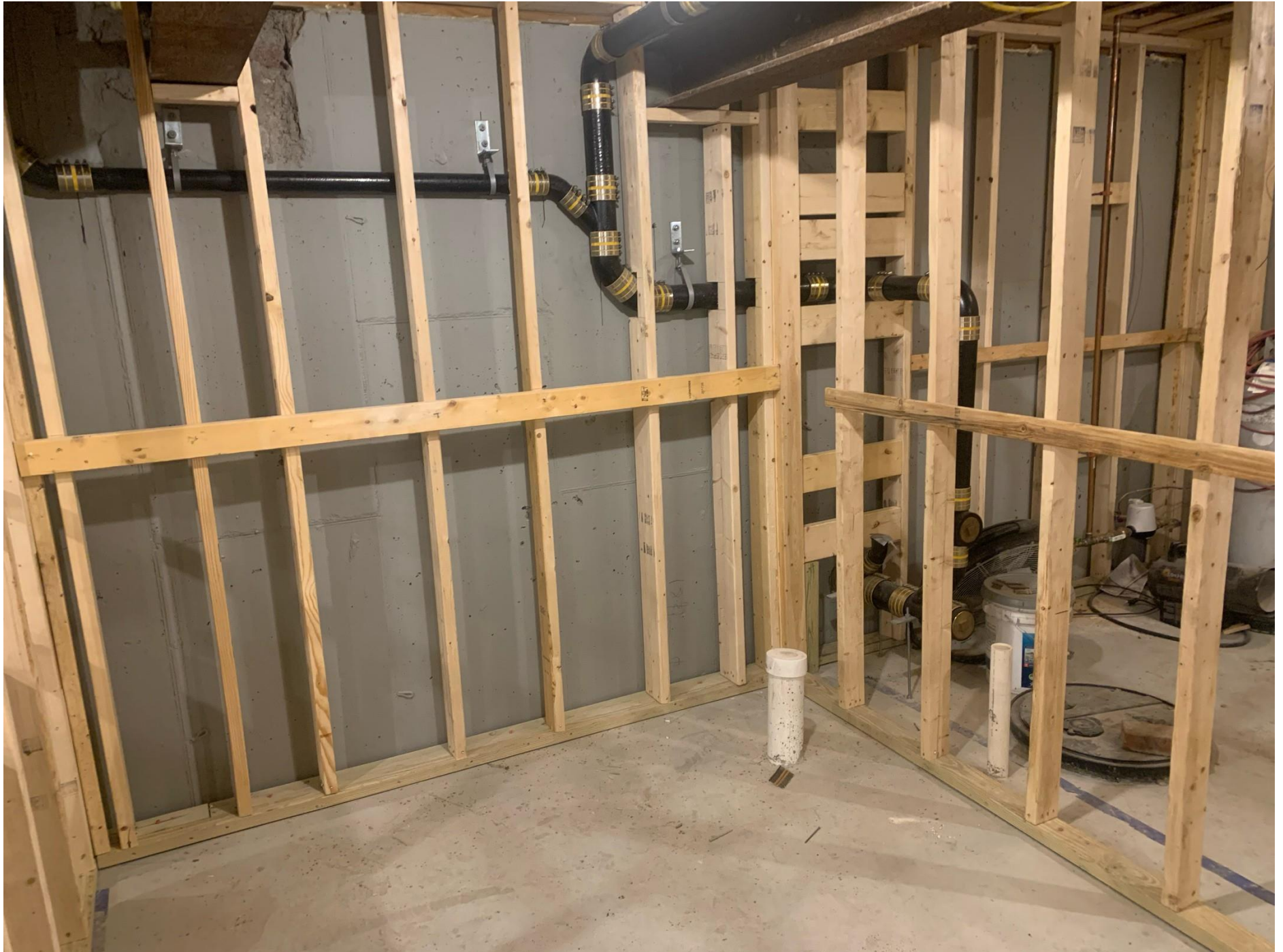
Inside – Level 1 – Garden Level – ADA Compliant Restroom 1
