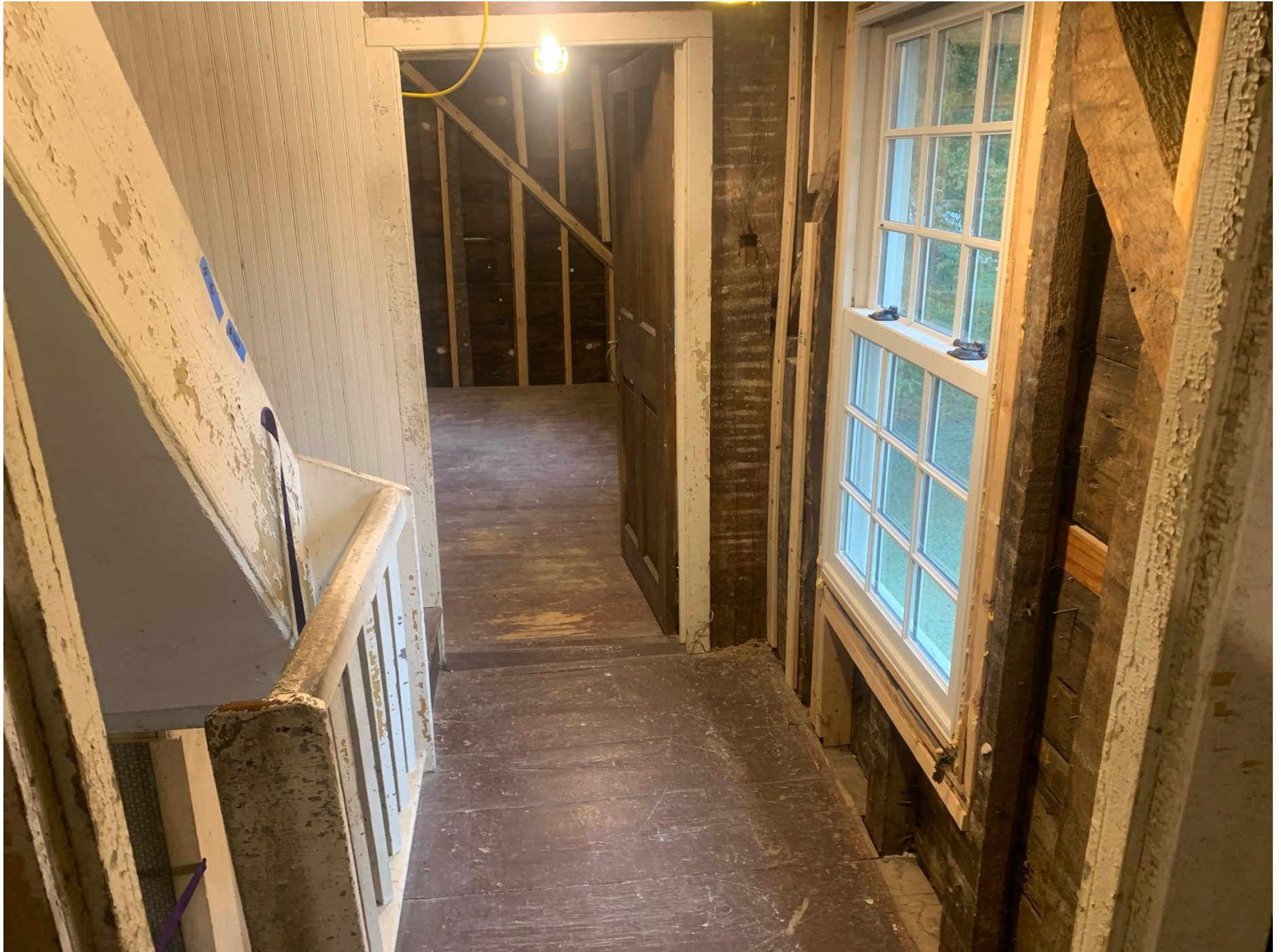
Inside – Level 3 – Second Floor – Front Hall – West to East
