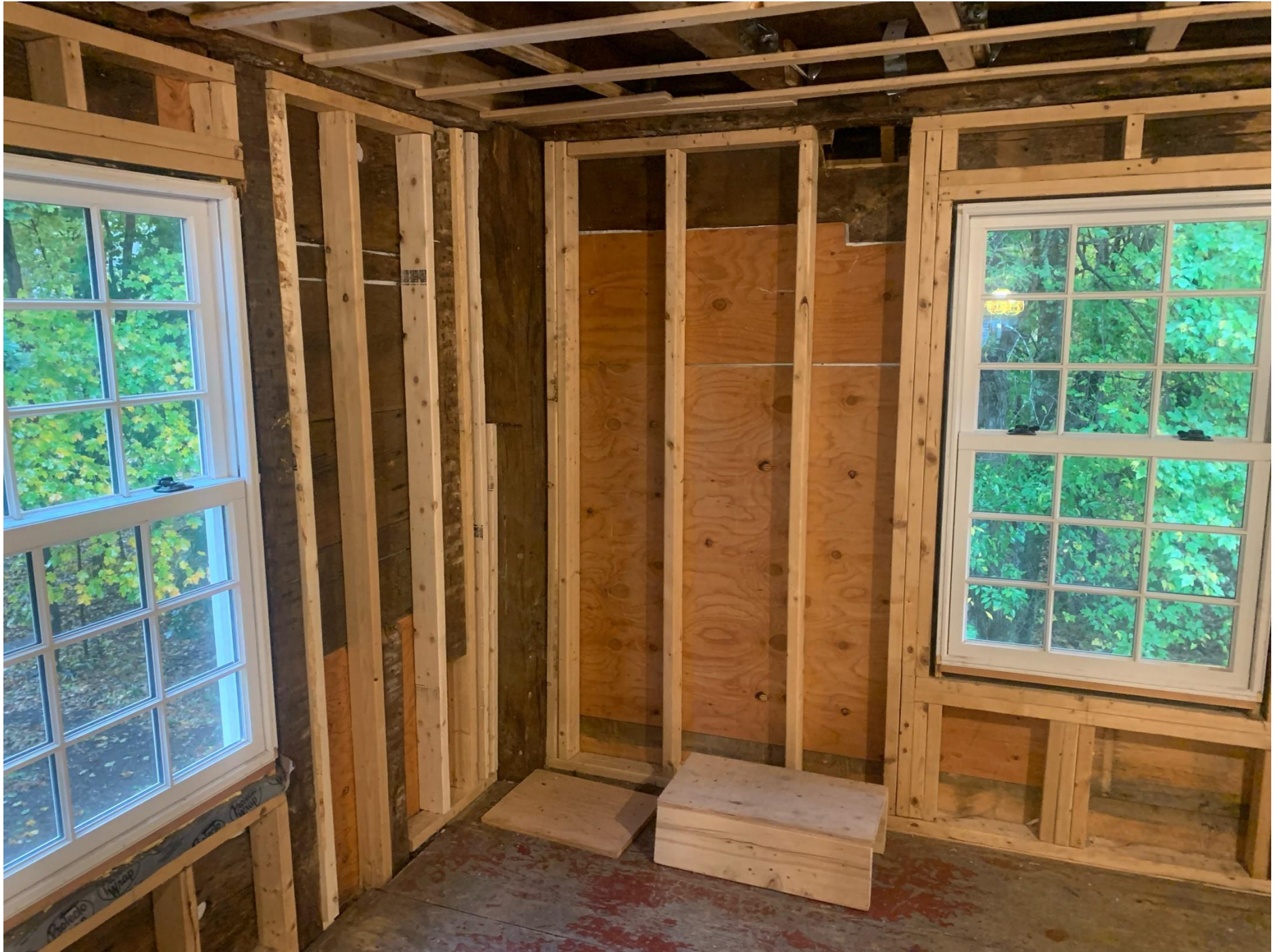
Inside – Level 3 – Second Floor – PracUce Room B
