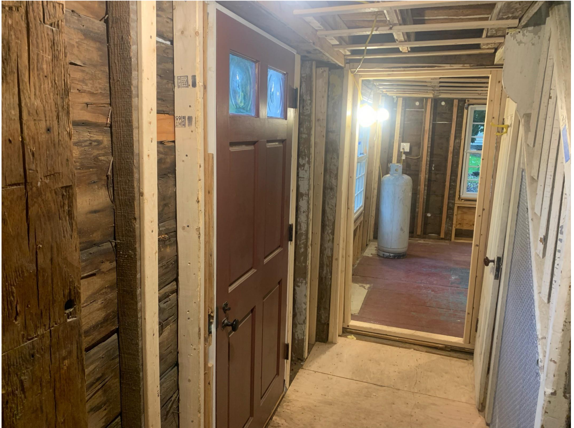
Inside – Level 2 – First Floor – Front Hall – West to East
