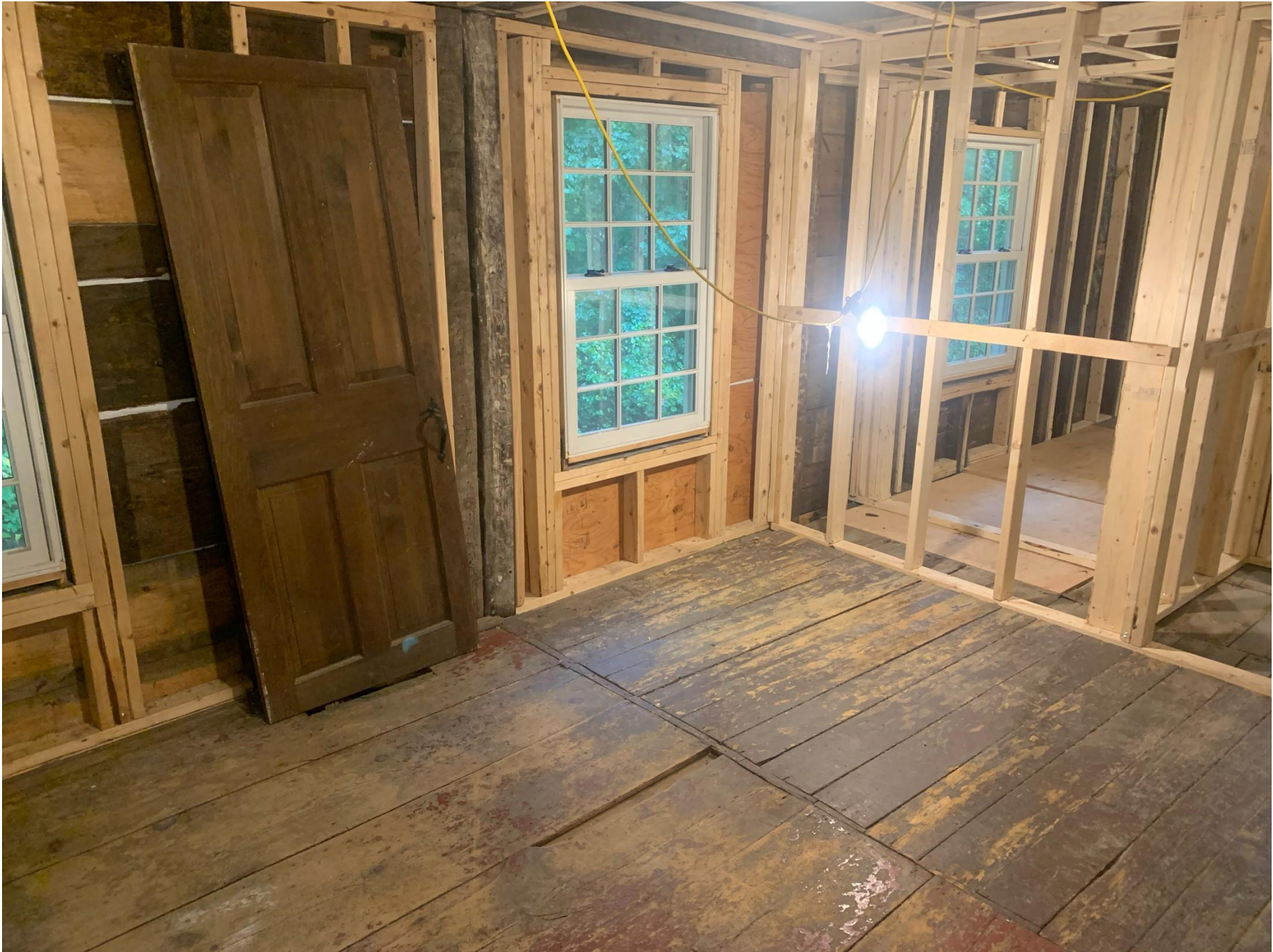
Inside – Level 3 – Second Floor – PracUce Room B
