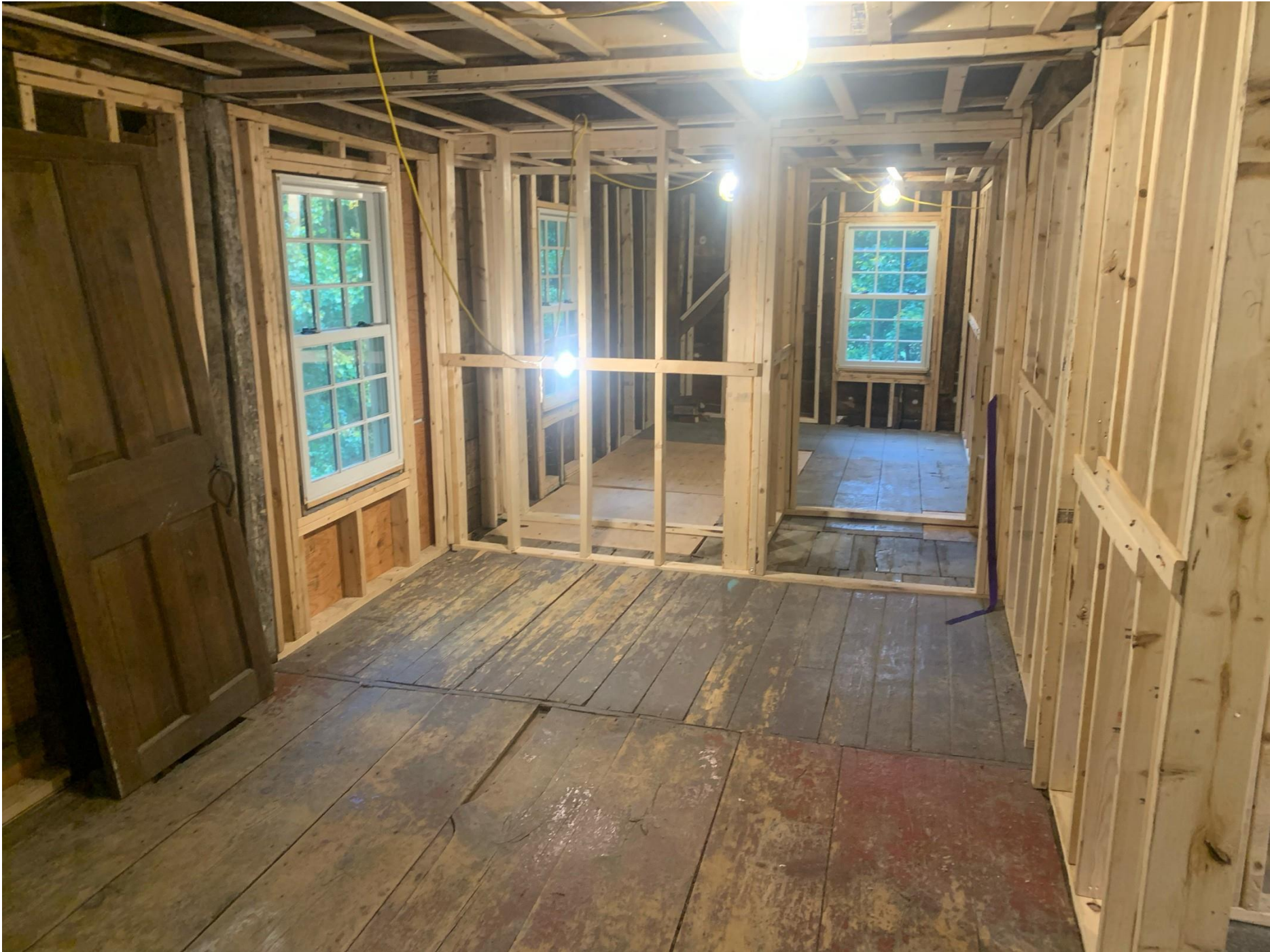
Inside – Level 3 – Second Floor – PracUce Room B
