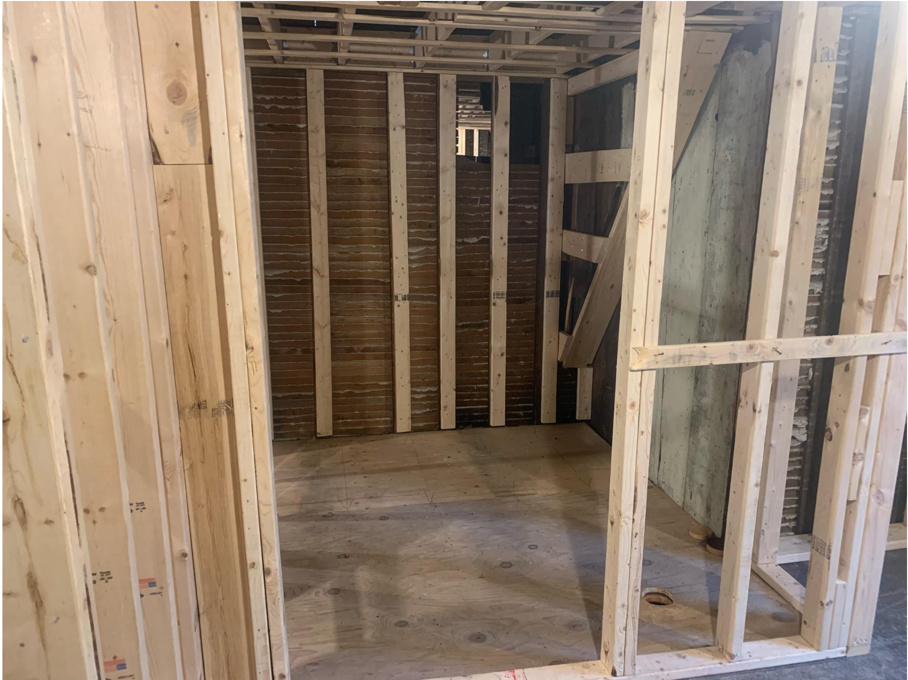
Inside – Level 3 – Second Floor – ADA Compliant Restroom 3
